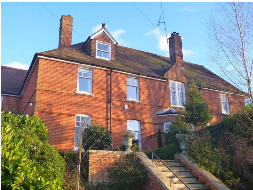
Fig. 49: North View and South View (east side) – Category 1
