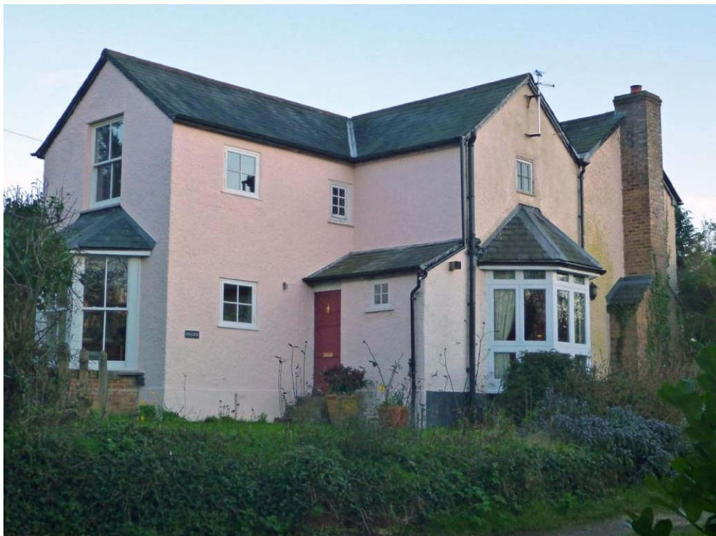
Fig. 37: Hillside (south side) – Category 1 C19th detached house. L-plan with a gable chimney stack. It is built in an imposing position overlooking the road. Good 2 over 2 sashes to bay on the front elevation.
