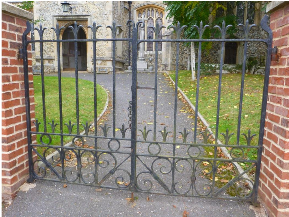
Fig. 52: Wrought iron gates outside the Church of Saint Mary the Virgin.
