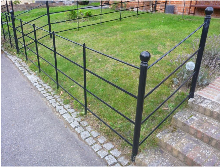
Fig. 53: Slender Estate fencing outside Lodge Farm Cottage and Blacksmith's Cottage
