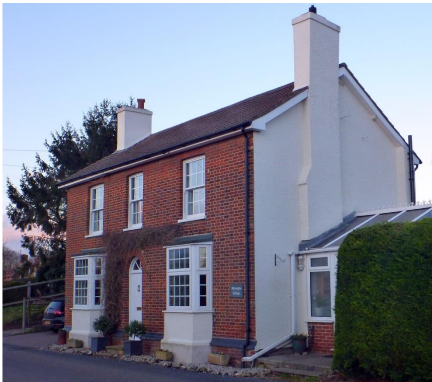
Fig. 39: Millwrights Cottage (east side) – Category 2
