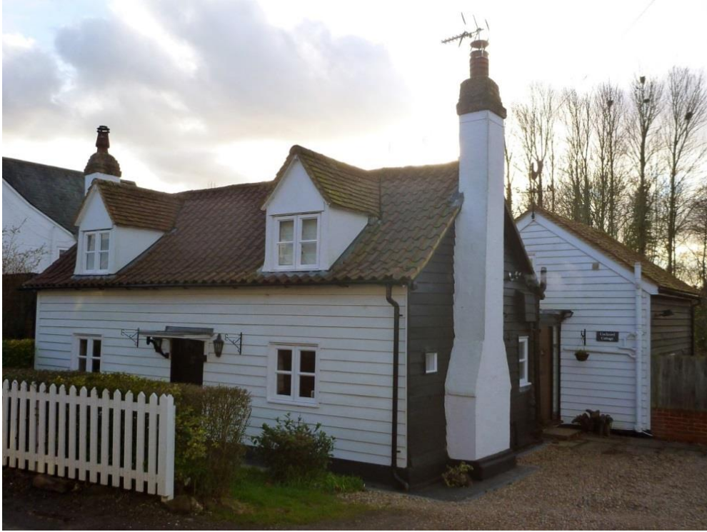
Fig. 17: Cock House (recently known as Cockerill Cottage) C18th cottage, weather-boarded with a pantiled roof. Ground floor and attics, with two tiled gabled dormers, two gable chimney stacks. Weathervane at rear.
