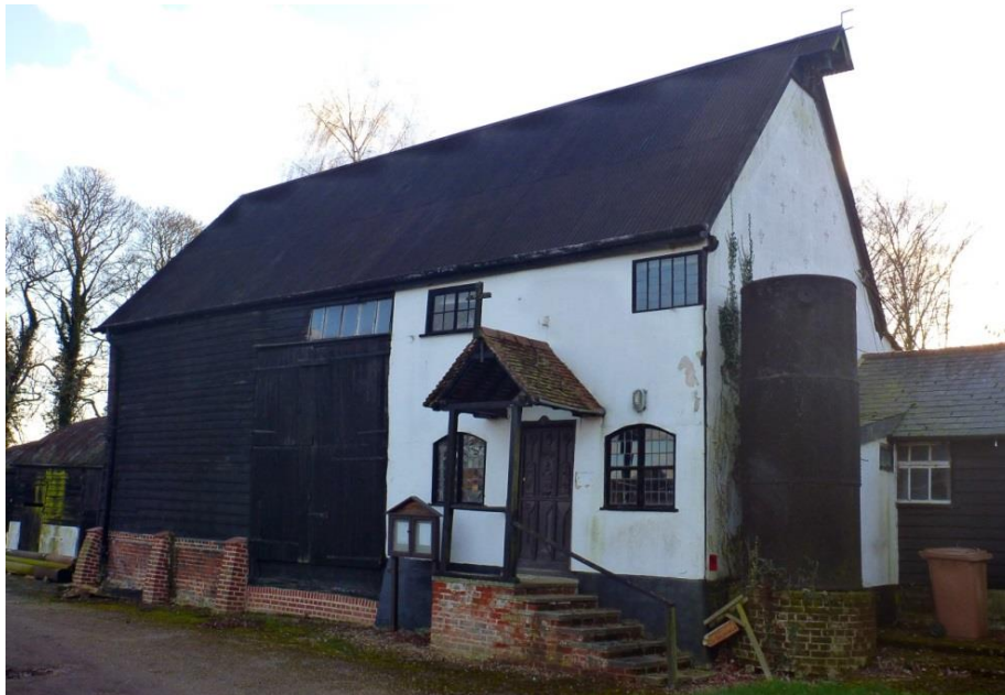
Fig. 24: Barn at Tinkers Hill Farm
