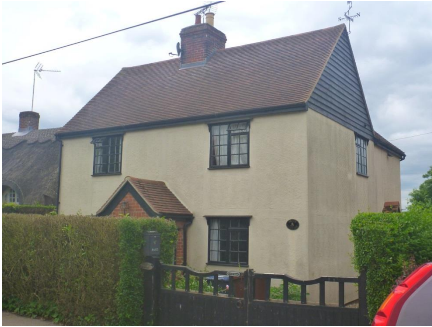
Fig. 40: Brook Cottage (west side) – Category 2 House shown on C19th historic maps now much altered. Rendered walls, weather-boarded side gables, tiled roof with a weathervane at the North end, and a central axial brick chimney stack. Modern front porch in brick with a tiled roof.
